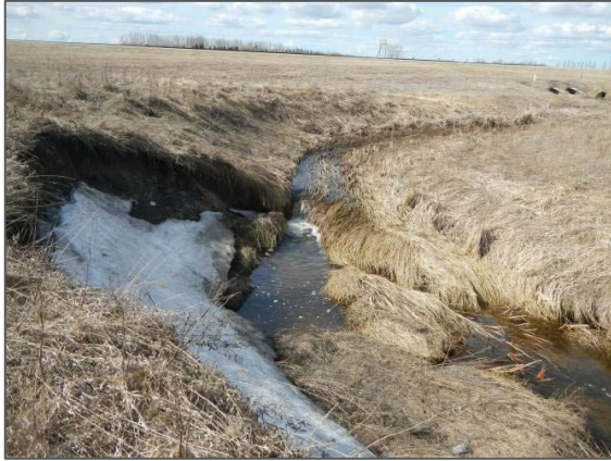
Figure 6-7. Erosion of Existing Channel
