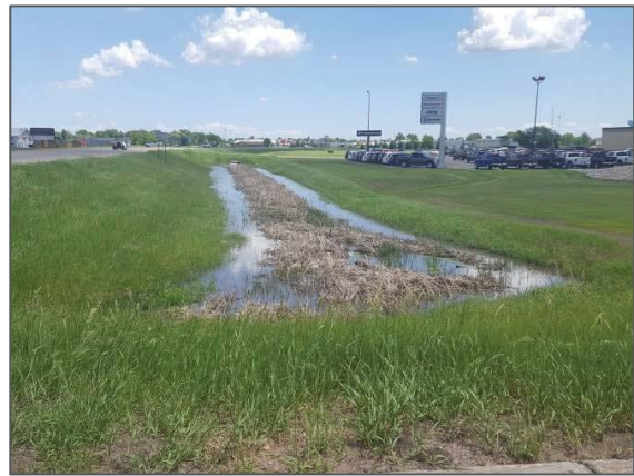
Figure 2-2. Excess Vegetation and Poor Grades Along CD 70
